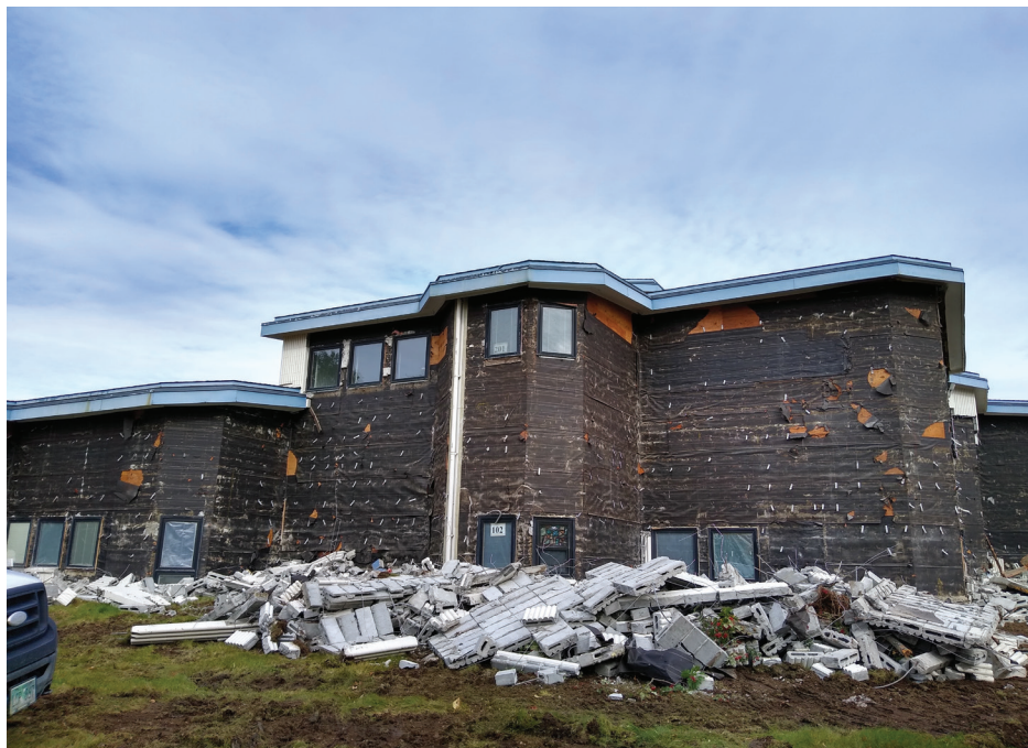
Figure 4. Removal of Masonry Veneer
