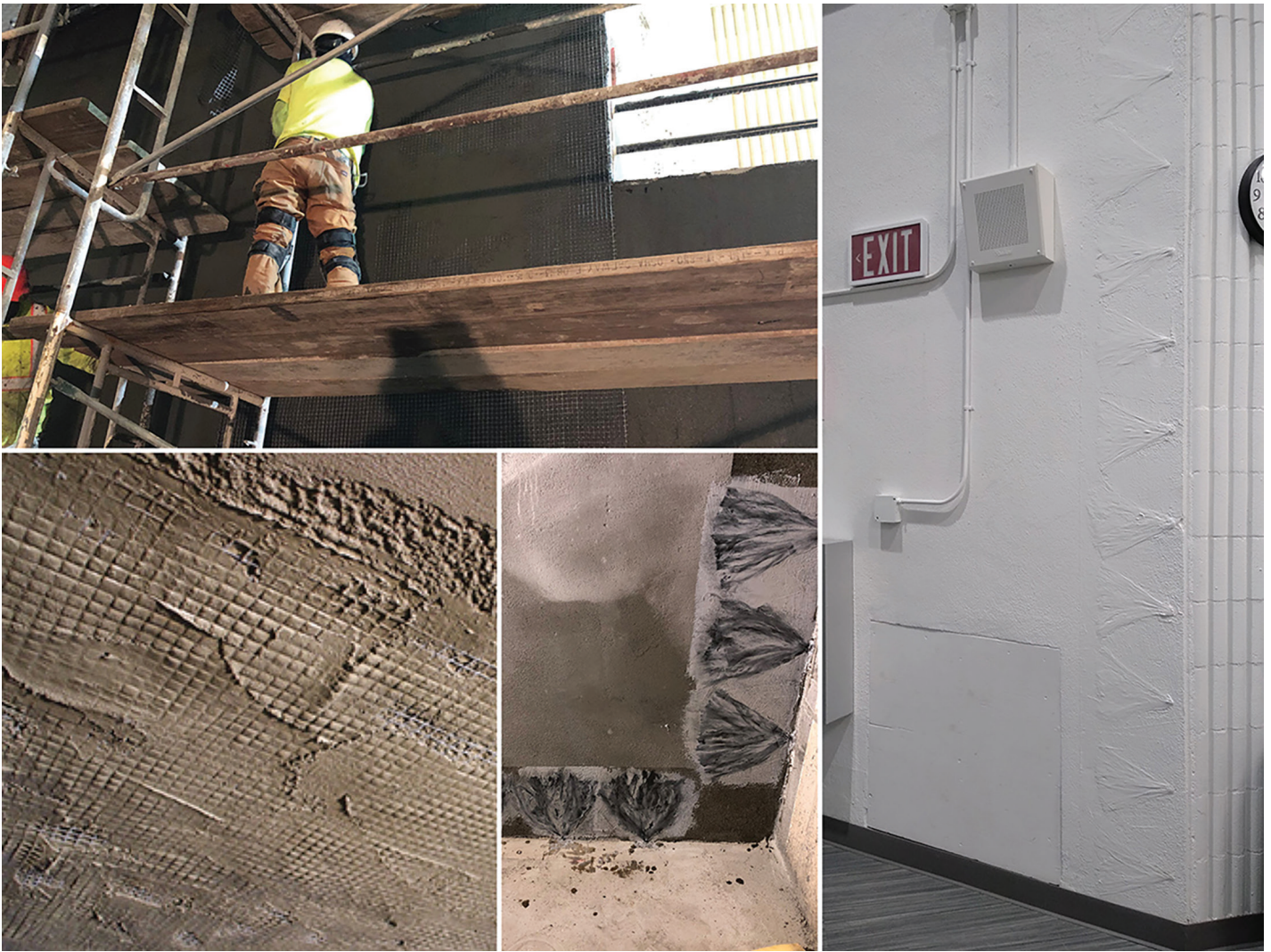
Figure 5. Fabric-Reinforced Cementitious Matrix (FRCM)
