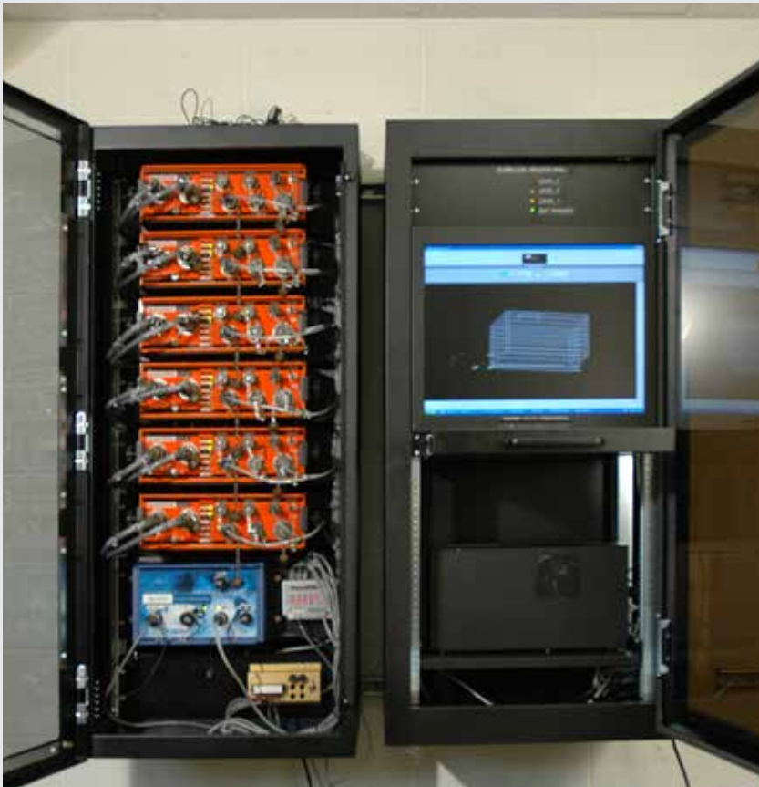
Seismic Monitoring System (SMS) provides real-time evaluation of the building response based on pre-engineered performance limits.
