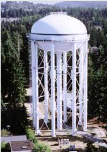
Renton Highland Water Tank Seismic Retrofit, Renton, WA
