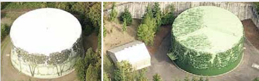
Sammamish Plateau Water Tanks 297 & 7MG
