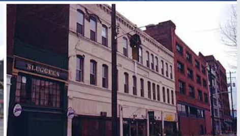
Nisqually Earthquake, Seattle - 2001
