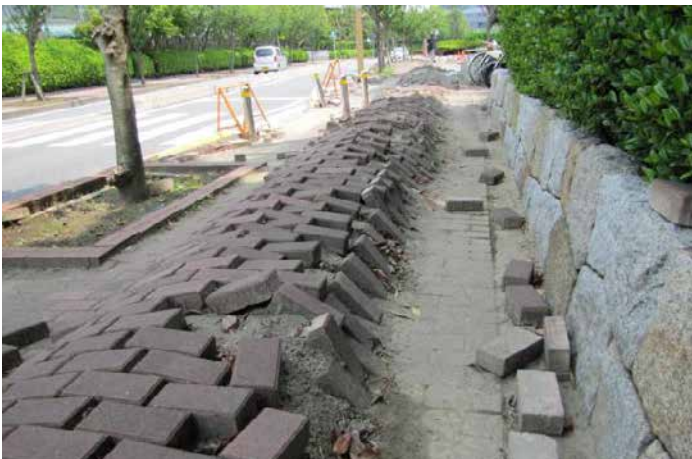
FIGURE 30 - Underground utility impacts (soil liquefaction) in Chiba (Tokyo metro) area. (Pierepiekarz)
