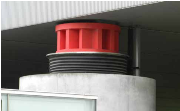
FIGURE 18 - Rubber seismic isolation bearing beneath a building in Tokyo. (Taylor)
