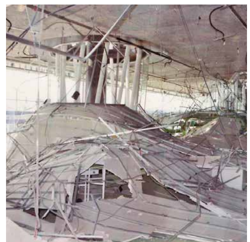
FIGURE 15 - Unbraced suspended ceiling collapse at the Sendai Mediatheque. (Siu)
