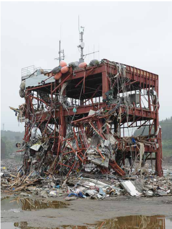
FIGURE 4 - Modern Disaster Prevention Center building in Minami Sauriku after the 14m high tsunami (Swanson)
