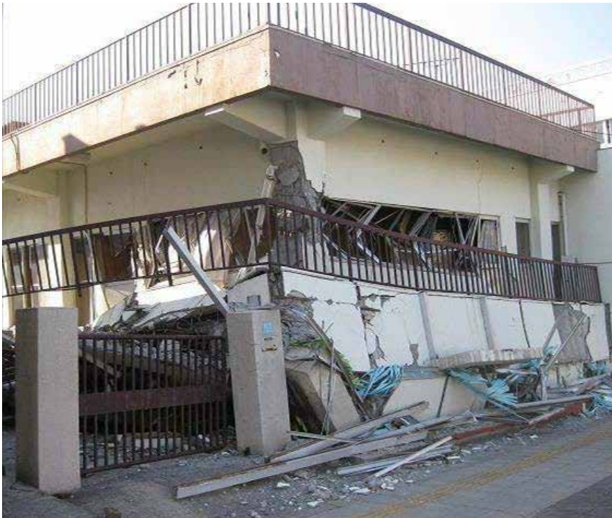
FIGURE 10 - Non-ductile concrete frame-over shear wall building. First-story walls failed in out-of-plane direction, Second-story columns failed in shear. (image courtesy of Motosaka)
