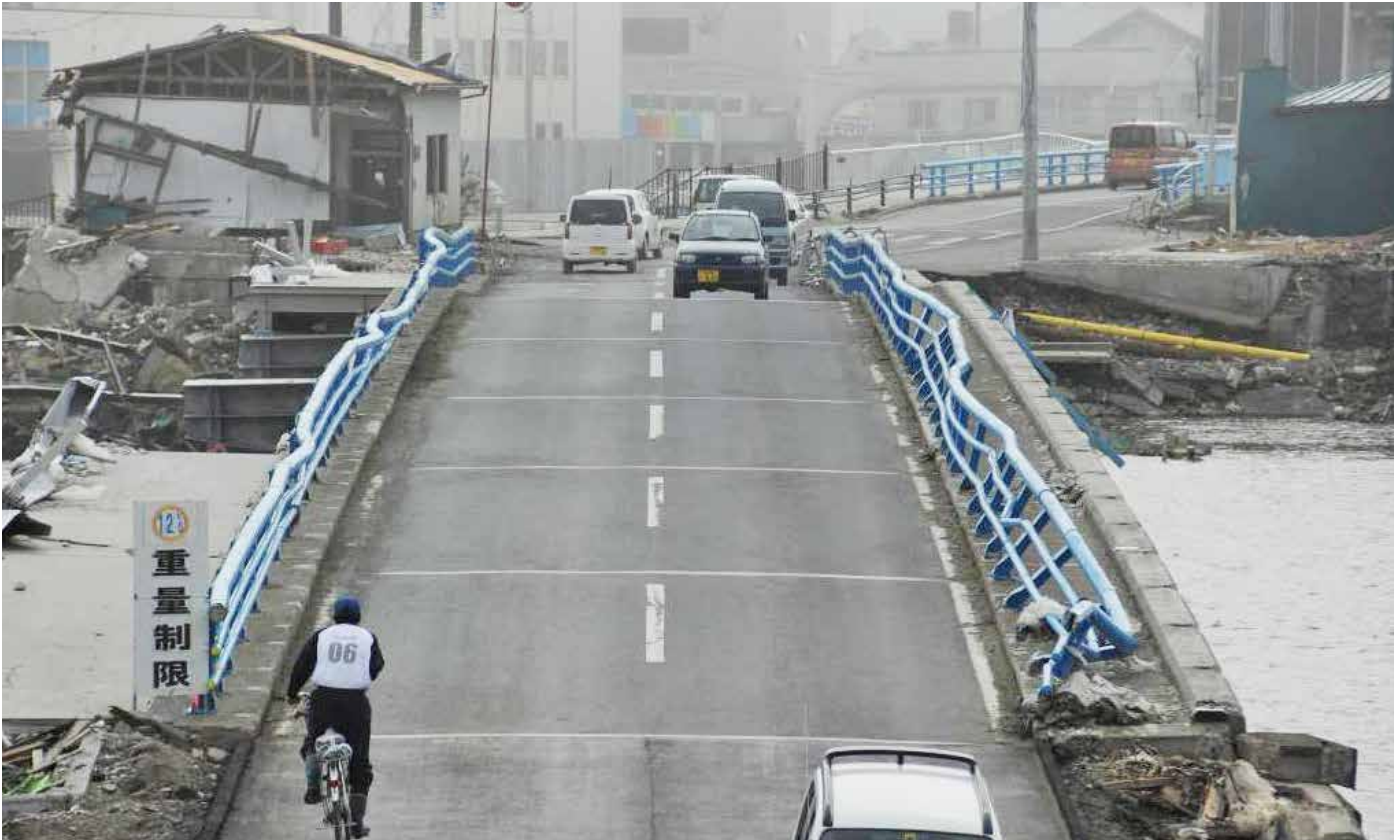
FIGURE 26 - Functional Low-Profile Vehicle Bridge In Ishinomaki City. Note Damage from Tsunami to Leading Edge of Bridge Walkway and Guardrail on the left side of the photo. (Swanson)
