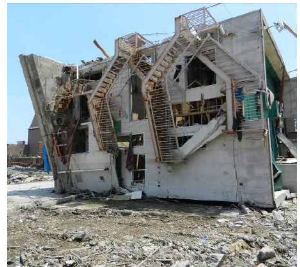
FIGURE 25 - Overturned steel-framed structure in Onagawa City. (Taylor)
