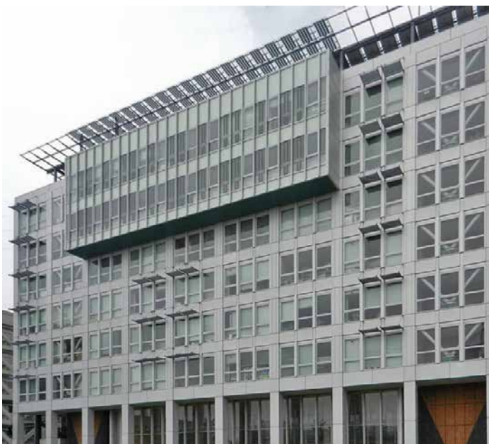
FIGURE 20 - Tohoku Institute of Technology Building with damping system for earthquake protection. (Taylor)
