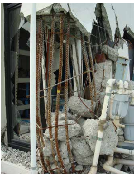
FIGURE 11 - Non-ductile shear wall boundary member detailing at a penthouse on top of a nine-story concrete building with a two-story podium. (Siu)
