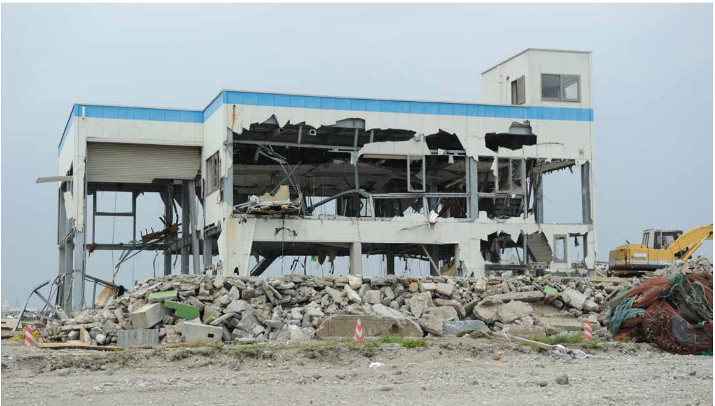
FIGURE 6 - Tsunami Damaged Steel Moment Frame Building in Natori from 7m Tsunami Height (Swanson)
