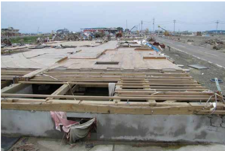
FIGURE 24 - Destroyed wood-framed buildings in Arahama Ward (Sendai). (Pierepiekarz)
