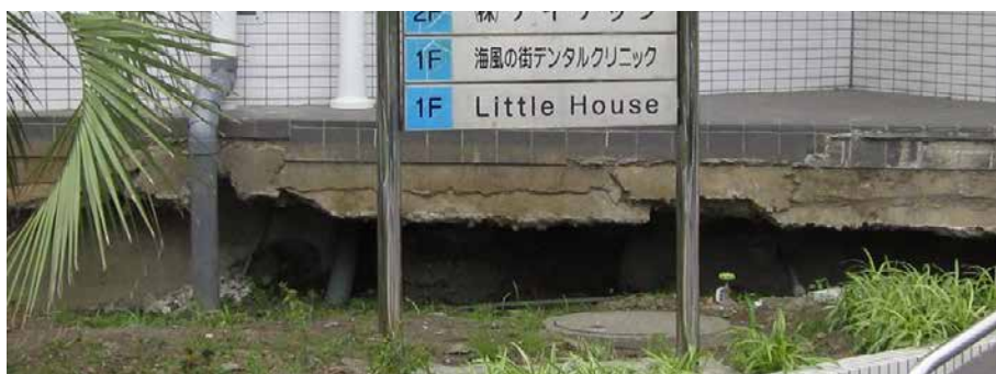
FIGURE 9 - Temporary utility connection following settlement caused by liquefaction in Urayasu City (Lindquist)
