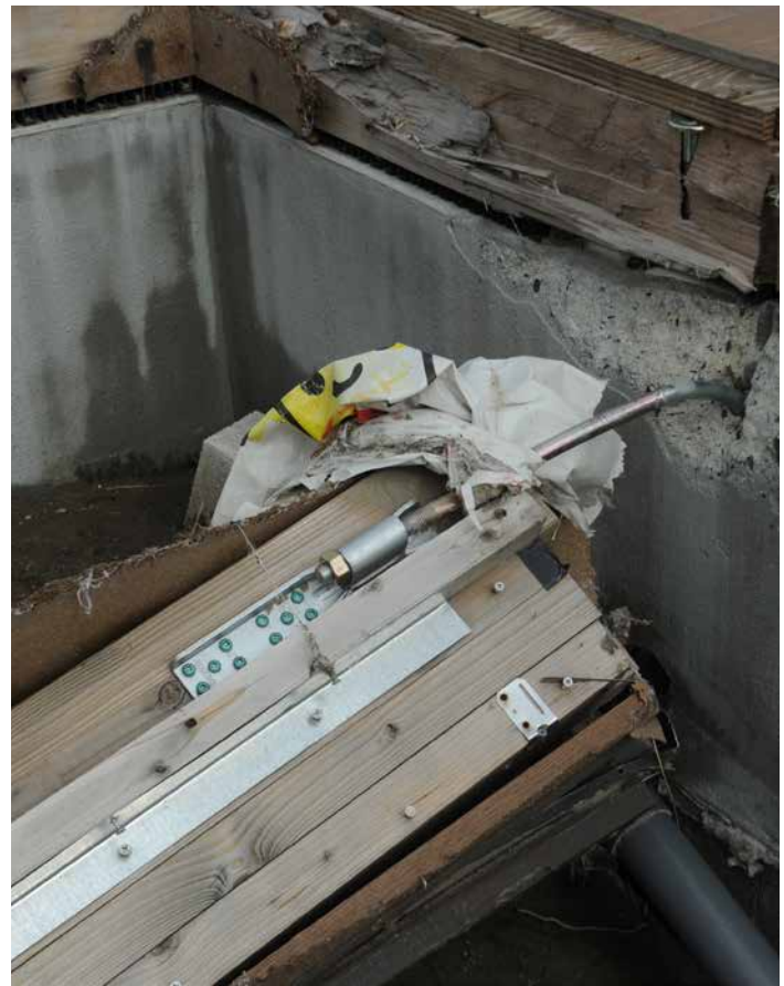
FIGURE 5 - Bent Wood-framed Shear Wall Hold-Down Connection from Tsunami (Swanson)
