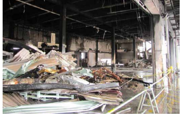
FIGURE 29 - Fire-following-earthquake impacts at Sendai Airport cargo area. (Pierepiekarz)
