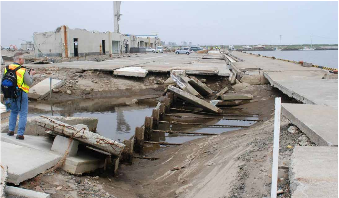
FIGURE 27 - Waterfront Tsunami Scour Behind Seawall in Yuriage. Note Exposed Seawall Tiebacks. (Swanson)
