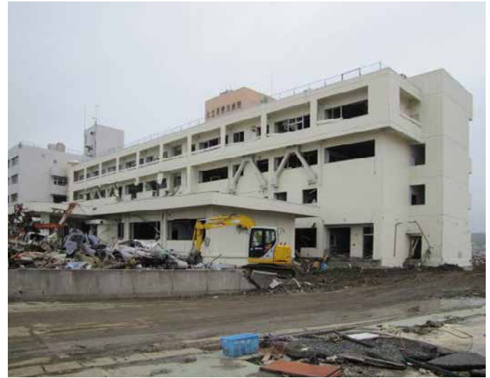
FIGURE 23 - Retrofitted hospital in Minamisanriku Town survived the ground shaking and provided shelter from 15m tsunami. (Pierepiekarz)
