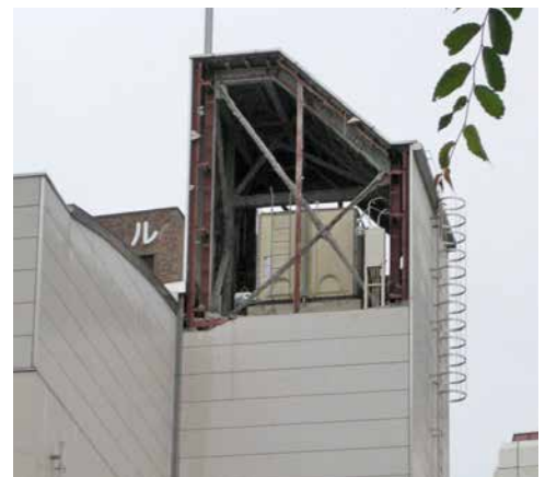
FIGURE 14 - Cladding damage at a school in Sendai. (Siu)
