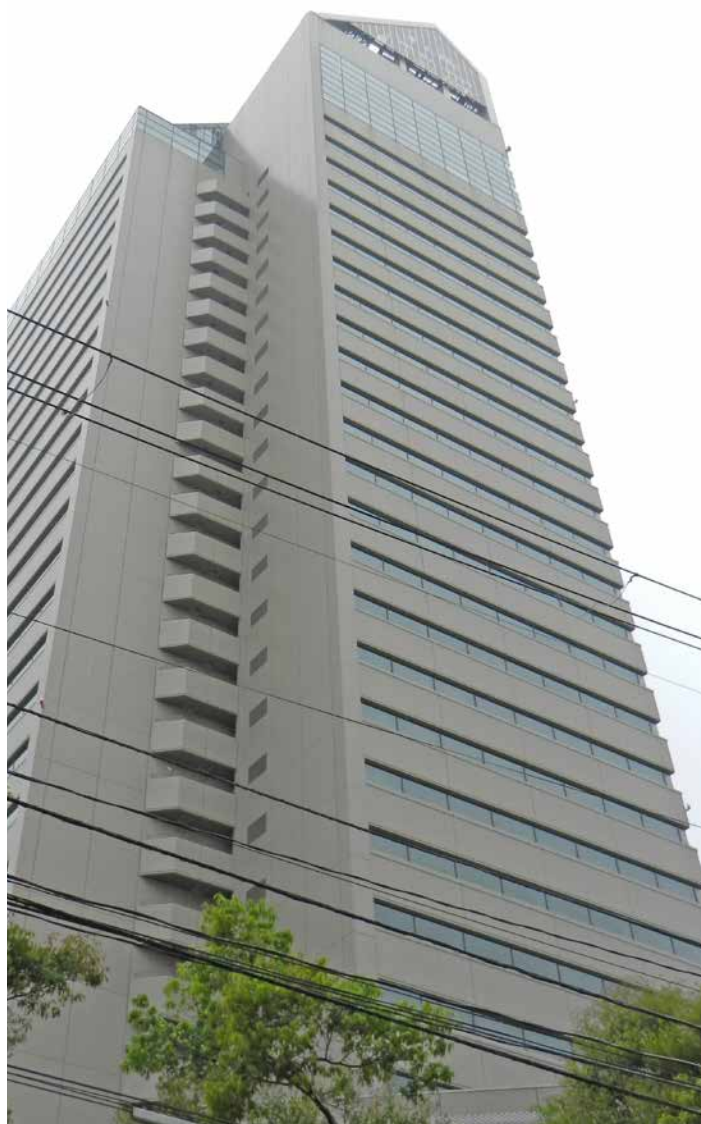
FIGURE 16 - High-rise building in Sendai. No structural damage was reported, but businesses and equipment on the top floors were damaged. (Taylor)
