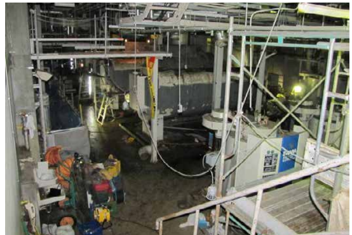
FIGURE 31 - Sendai Airport – main utility room located below grade was flooded. (Pierepiekarz)
