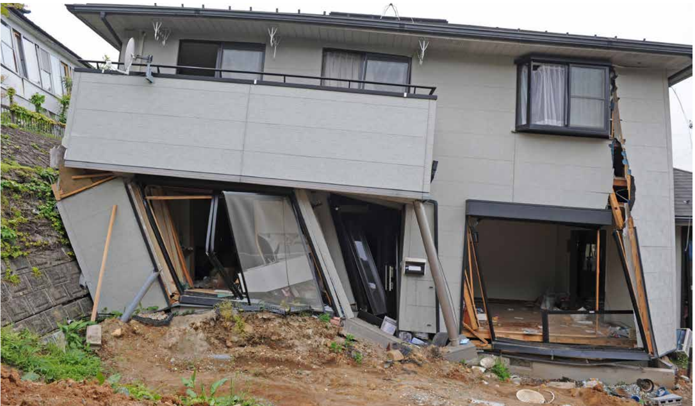
FIGURE 3 - Residential Building Collapse from large areal landslide beneath a residential neighborhood in Sendai City, Aoba Ward (Swanson)
