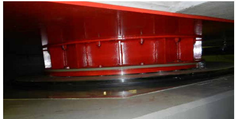
FIGURE 19 - Sliding seismic isolation bearing beneath a building in Sendai. (Taylor)
