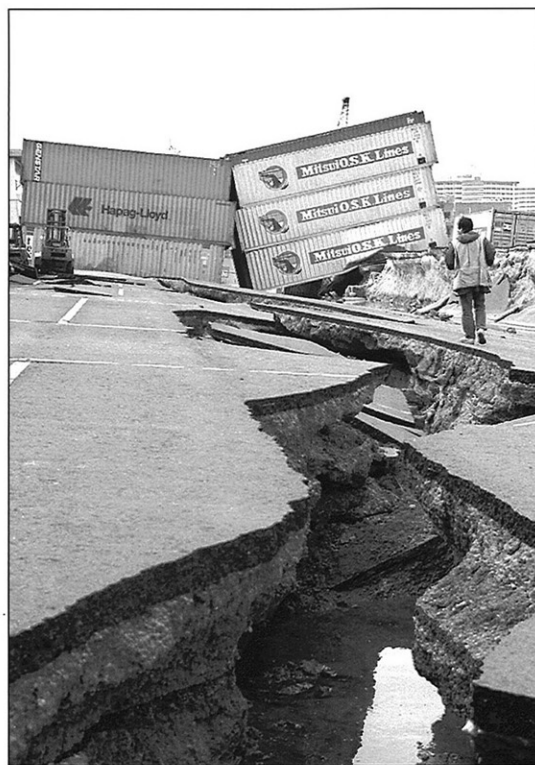
Damage from the magnitude 6.9 earthquake in 1995 crippled the Port of Kobe for years.
