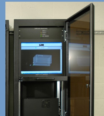
Seismic Monitoring System (SMS) provides real-time evaluation of the building response based on pre-engineered performance limits.
