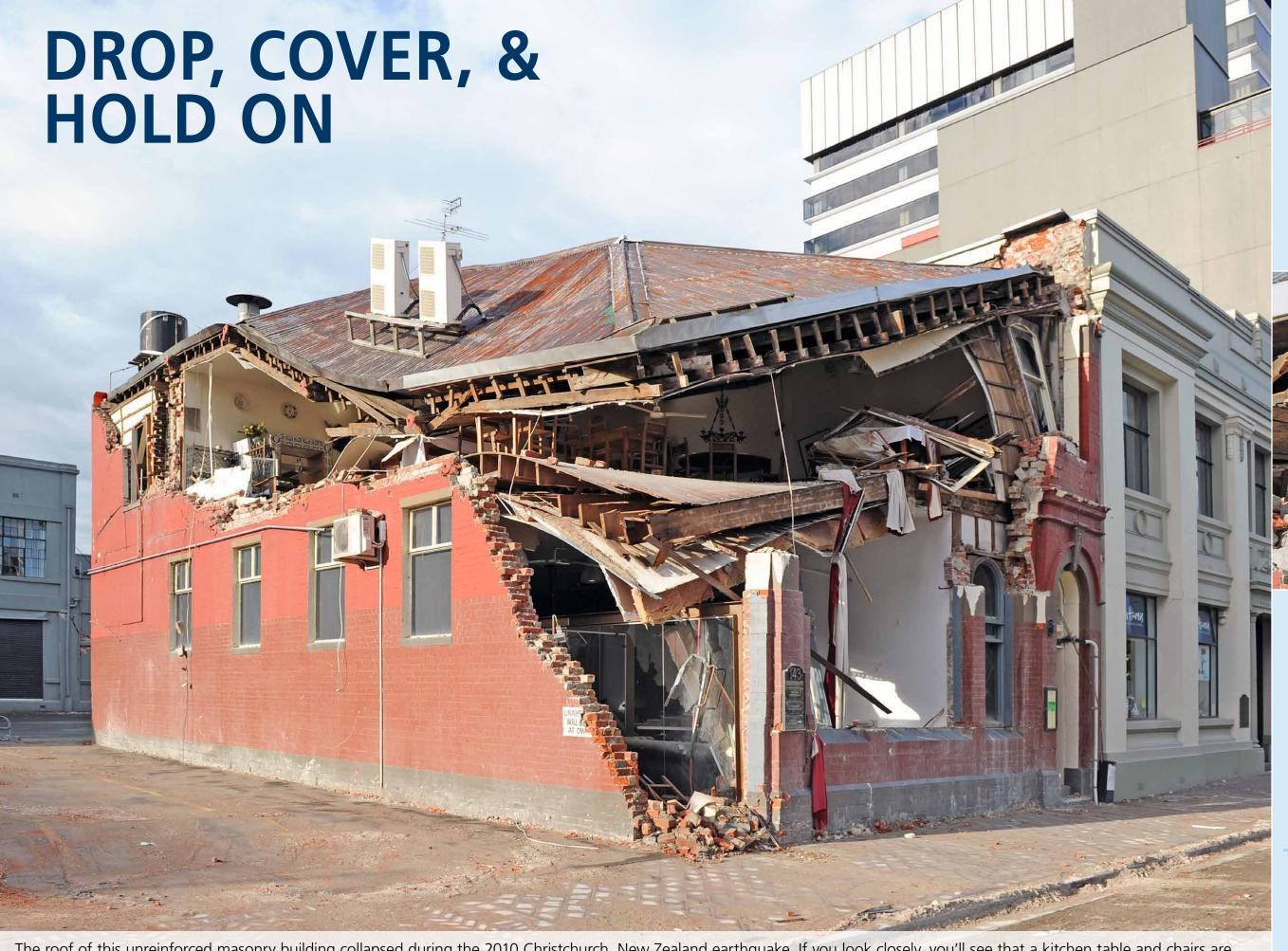
The roof of this unreinforced masonry building collapsed during the 2010 Christchurch, New Zealand earthquake. If you look closely, you'll see that a kitchen table and chairs are supporting the collapsed roof, illustrating that the safest place to be during an earthquake is under a sturdy table or desk.
