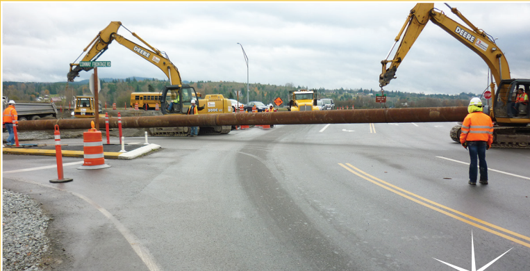
Roundabout sleeve line installation
