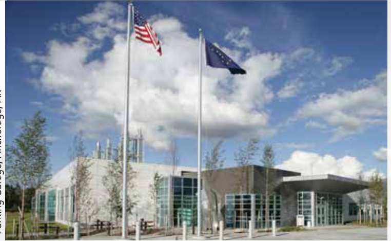
Providence Alaska Medical Center Parking Garage, Anchorage, AK
